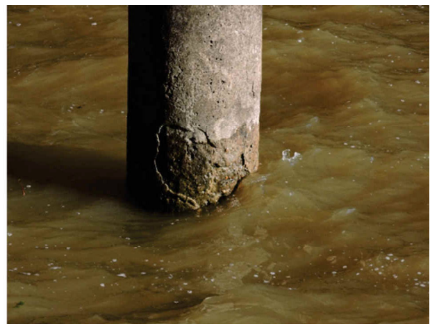
Figure 2. Detail of a column.
