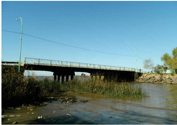
Figure 1. Bridge over the Villa Elisa channel at Boca Cerrada, Punta Lara.
