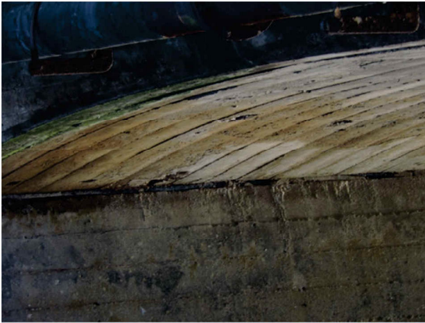
Figure 3. Detail of the orange staining cause by metal oxides.
